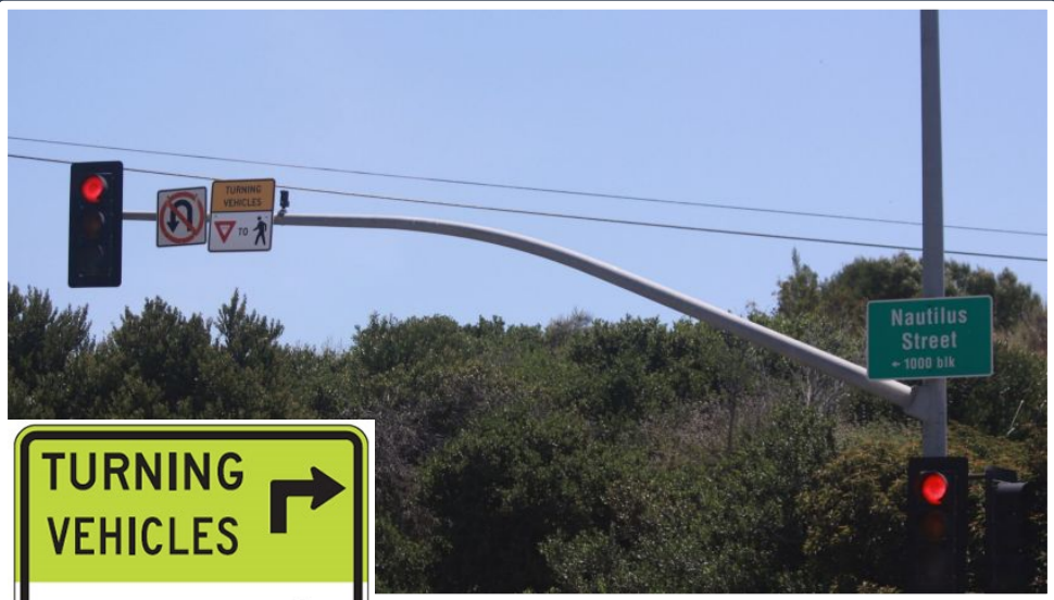
Mast-arm mounted “TURNING VEHICLES YIELD TO PEDESTRIANS” signs on George Griffith Boulevard
